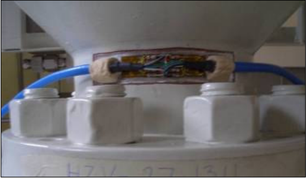
FIGURE 6 Installed Strain Gauges
