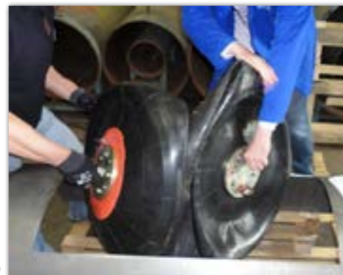
Air-bag insertion through pipe aperture
