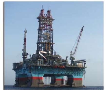
Maersk Developer Rig
