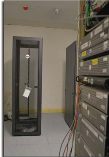
Glenugie Upgrade in Progress
