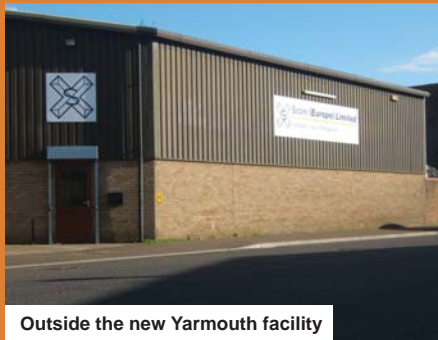
Outside the new Yarmouth facility
