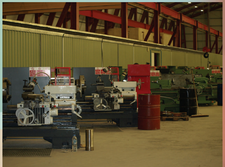
The new machine shop at shed 2
